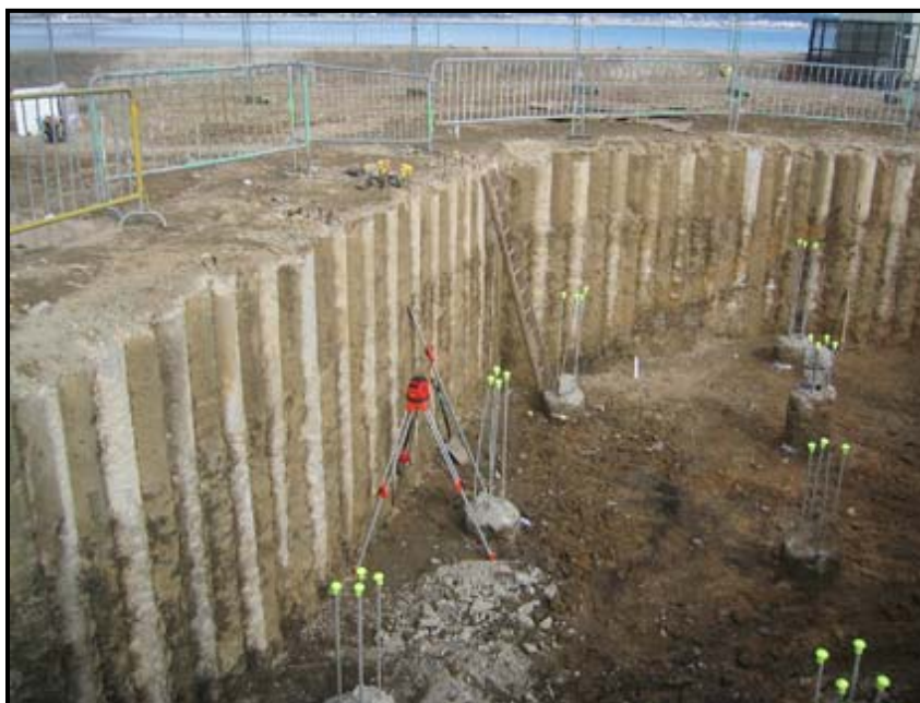
(اجرای شمع (Bored pile walls))
